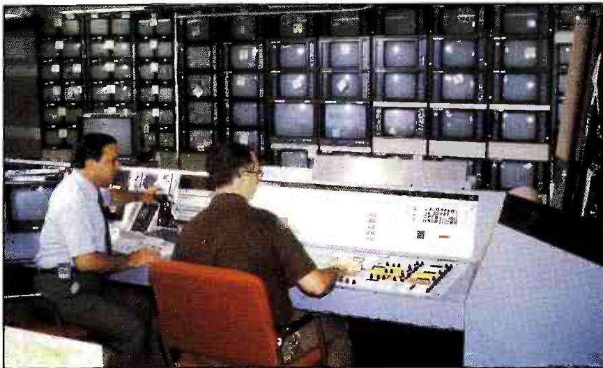
ABC's master control room is being built on wheels. It will consist of four 40-foot containers that will be driven into The Round-Up Centre and set up, eliminating major assembly on-site.
