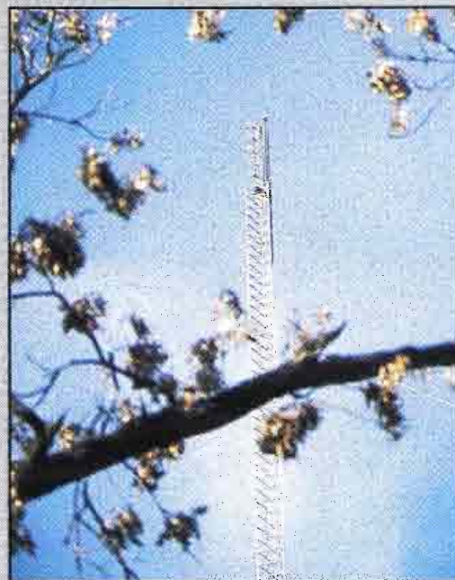
The tower was officially accepted on Feb. 27, 1987, 27 weeks after ground was first broken for the project. The tower inspection process was detailed and lengthy. All bolts were checked for tightness by a consultant for the station and by a consultant for the tower manufacturer.
