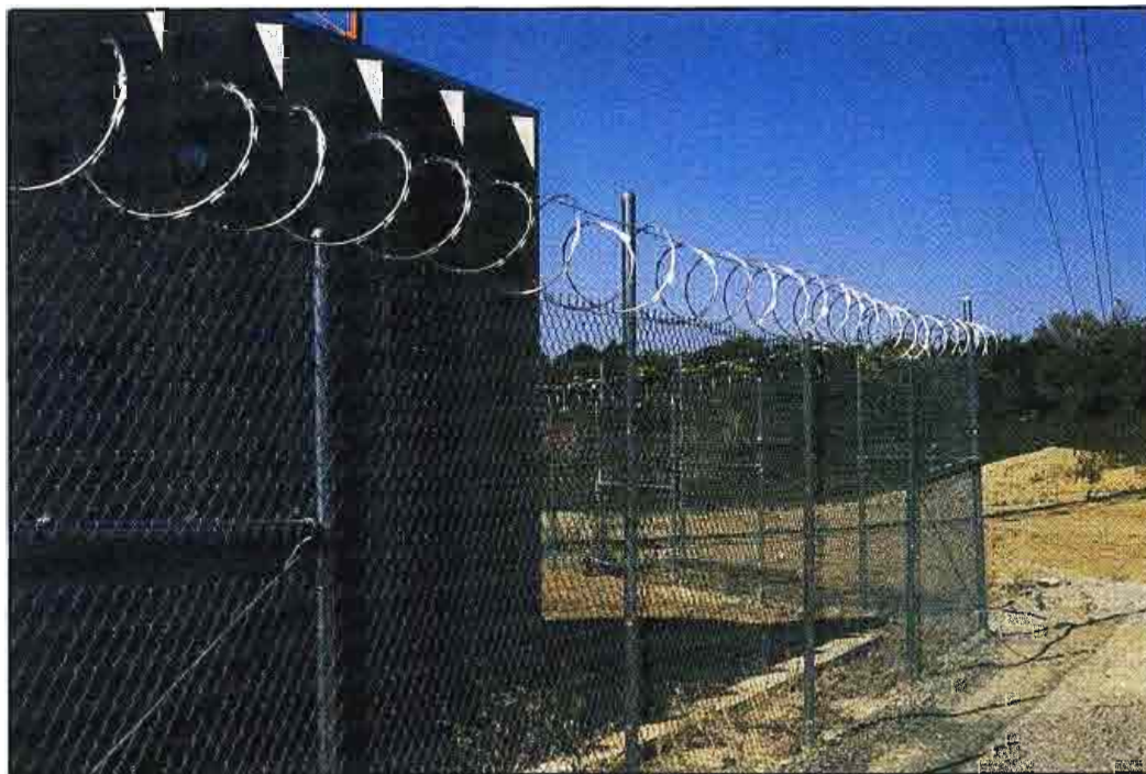
Security for the facility was an important design consideration because the site operates unattended in a remote area. Heavy-duty fencing surrounds the complex.
