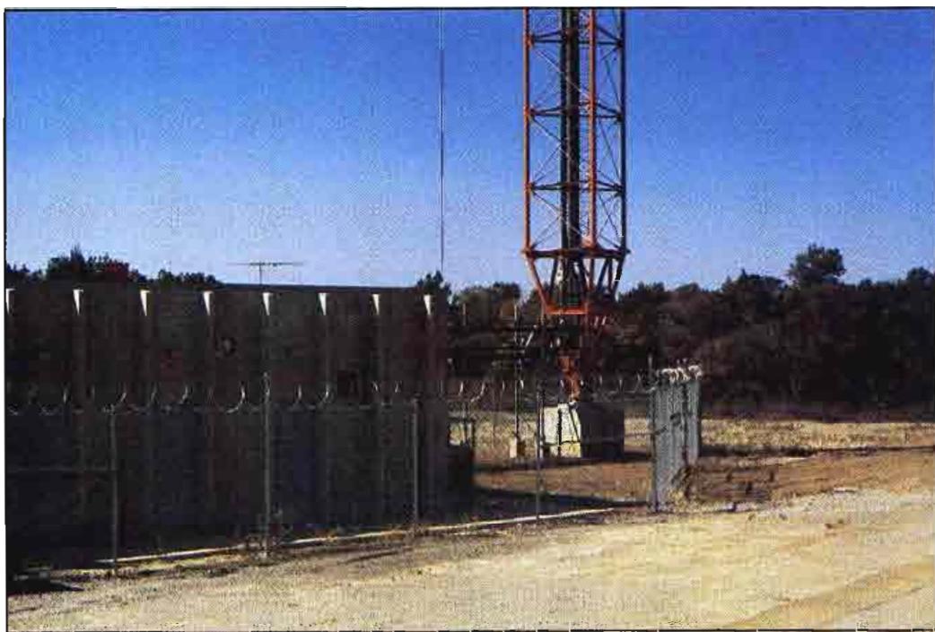
The KLSI community tower site is located east of downtown Kansas City, MO. The 1,024-foot tower and 3,024-square-foot building provide transmission facilities for four Class C FM stations and up to 20 2-way radio systems.
