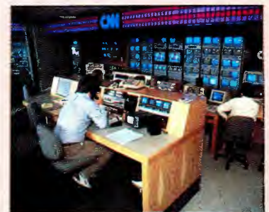
One of the control rooms for the Cable News Network. The facilities operate 24 hours a day, seven days a week.
