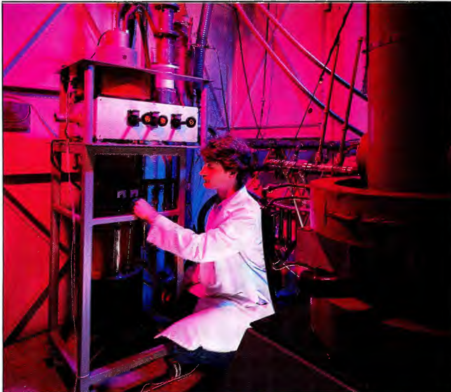
After years of development, the Klystrode is on the air in regular TV service. In a pioneering move, the Georgia Public Television system has placed in service two Klystrode-equipped transmitters. With those installations, the Klystrode moves from the lab to the field. A Klystrode is shown undergoing final tests before shipment. (Photo courtesy of Varian EIMAC.)
