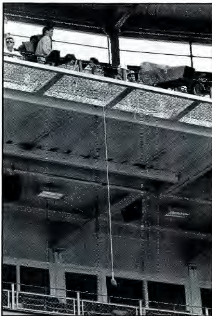
One of two suspended microphones used as primary crowd noise pickups for a baseball game.
