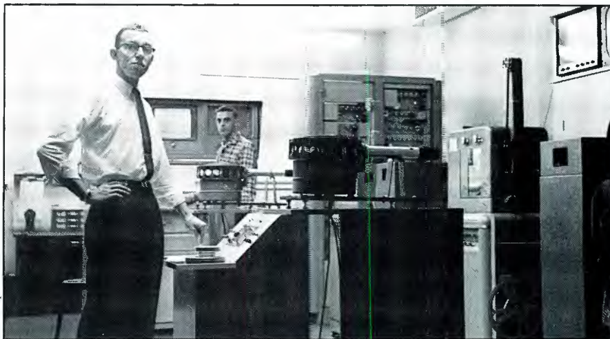
Film chains, such as the one shown here, were commonplace 30 years ago. Today, a TV station may have only one, and seldom use it. This photo of a portion of the WNED-TV, Buffalo, NY, master control room was taken in 1960. The station's Ampex VR-1000B tape machine can be seen in the background.
