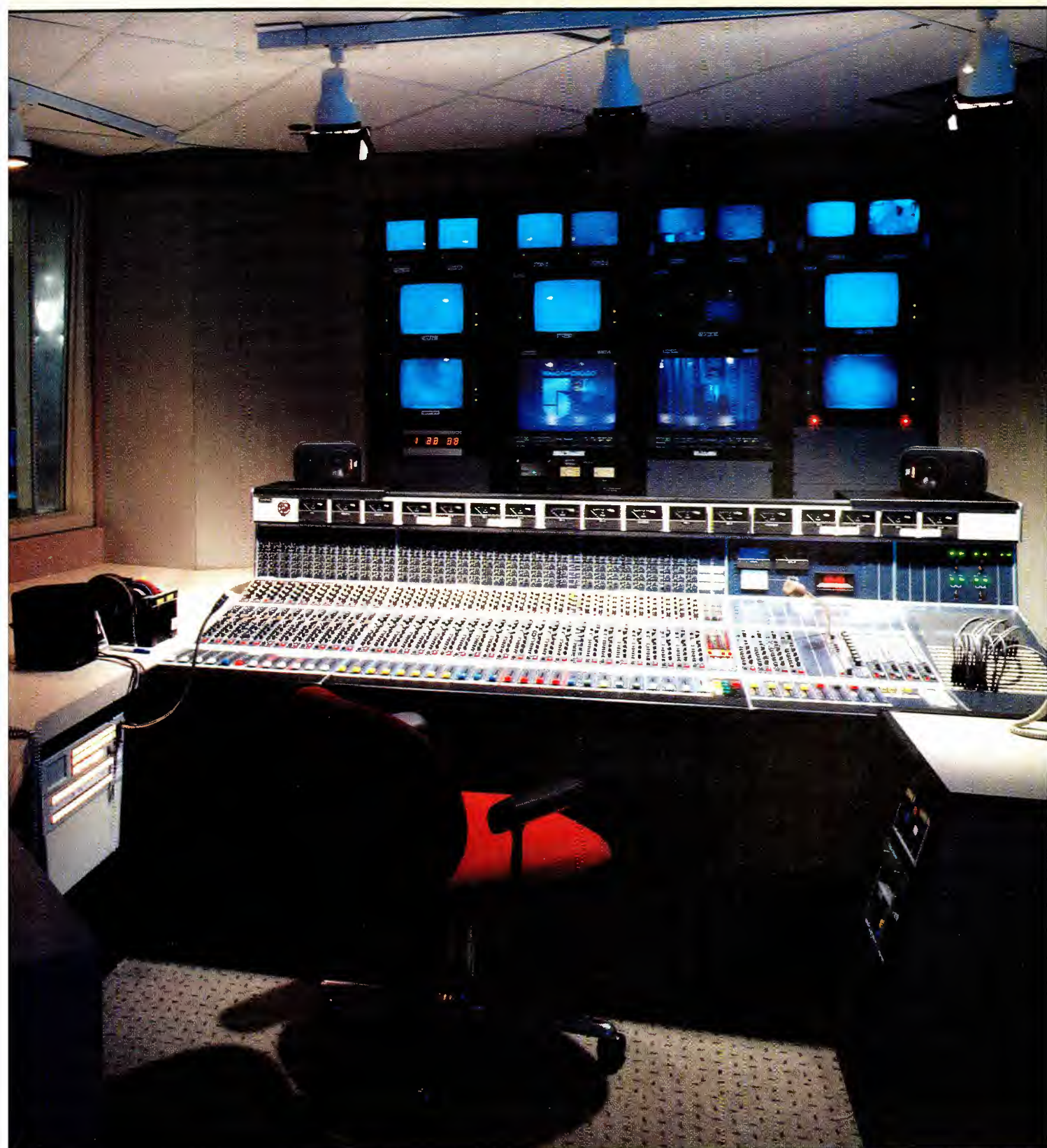
Audio control room in Chicago's recently relocated WMAQ-TV.
