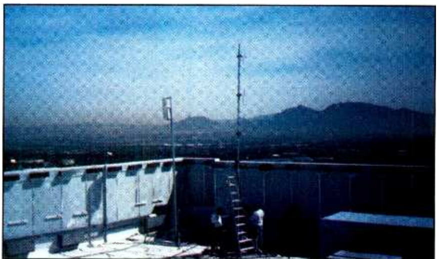
Eureka 147/DAB antenna (left) and FM comparison channel antenna on the roof of the Las Vegas Hilton for the first U.S. on-air demonstration during NAB '91.
