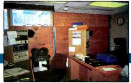
The WWRC newsroom was restored to service after wiping soot off the equipment and temporarily replacing heat-cracked windows with plywood. (Photo credit: Joseph Nunemaker.)
