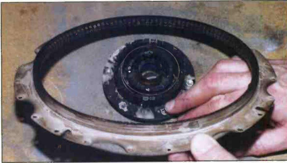
A contact ring and filament contact from one of the transmitters shows heat discoloration, tarnish and accumulations of dirt and grease due to environmental pollutants.
