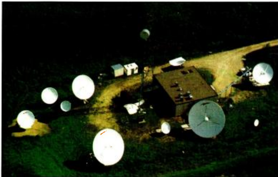
A station's satellite equipment can be a significant profit center if properly marketed. (Courtesy of Teleport Minnesota.)
