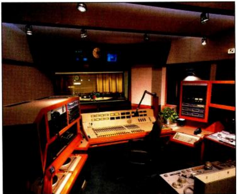
The modular installation of a control room and studio at WQXR, New York, shows that asymmetrical geometry and aesthetic interior acoustic finishes can both be accommodated.
