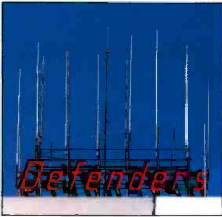
Stations take advantage of any high spot to mount RPU and 2-way antennas. This can set the stage for intermod problems.
