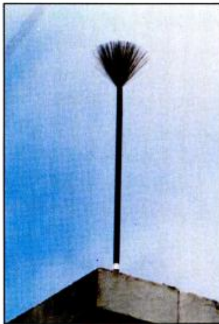
A static dissipation array consists of many air terminals with small point radii. These discharge ground charge, and build up the corona to discourage streamers.
