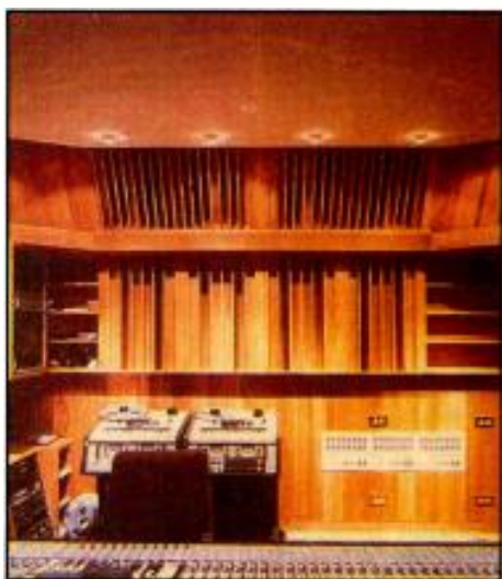
Diffusive rear wall in control room at Red Bus Recording Studio, London, features quadratic residue diffuser panels. (Courtesy of RPG Diffuser Systems.)
