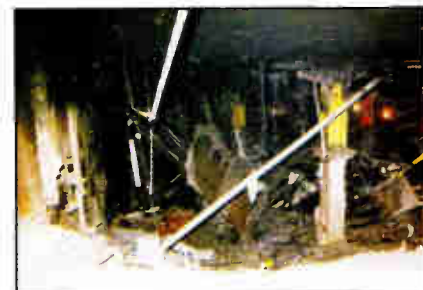
The crater from the terrorist bomb caused extensive damage to several floors in the underground parking garage. (Courtesy of AP.)
