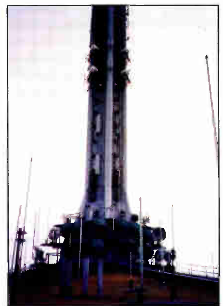
The roof of the World Trade Center provides the base of the multistation mast. The mast is located just above the 110th floor, which houses the transmitters for TV and FM stations.
