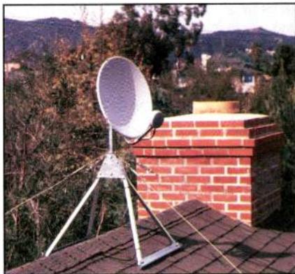
Roof-mounted receive dish for the Thomson/RCA DSS system. A rooftop location is not mandatory. Any location with unobstructed line-of-sight to the satellite can be used.
