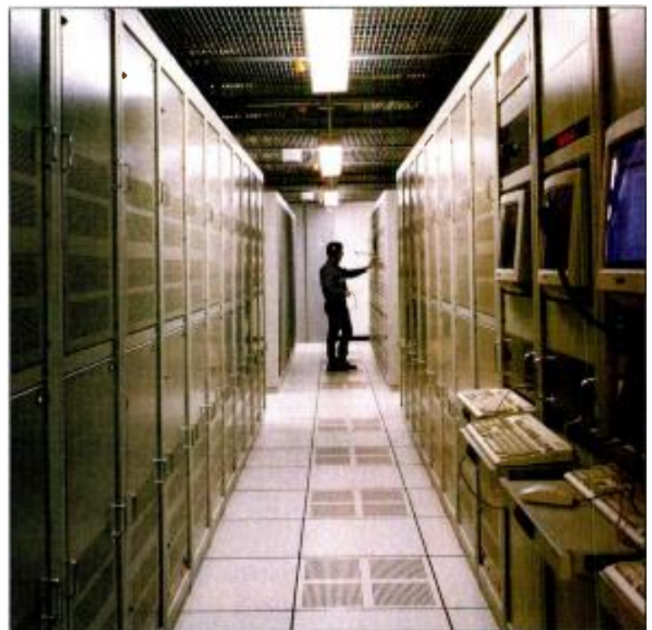
One of the newest facilities using serial digital technology is DirecTv, located in Castle Rock, CO. Several interconnected routing matrices provide serial digital signals throughout the facility. (Photo courtesy of Sony System Integration.)
