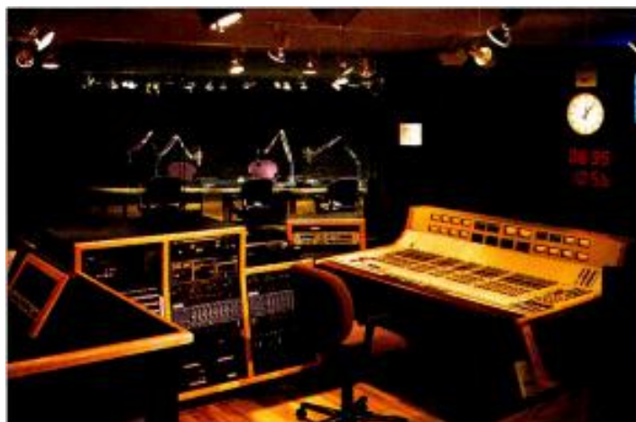
In National Public Radio's air control room for "All Things Considered" and "Morning Edition," careful shaping allows a large expanse of glass and improved air talent/production staff communication while maintaining an accurate monitoring environment. Monitor speakers (left, center, right) are mounted on point-loaded concrete pedestals.
