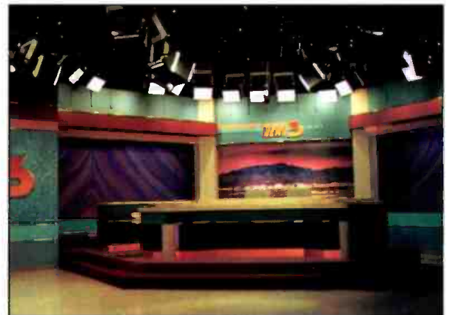
KVBC-TV, Las Vegas, installed the first focused VIDESENCE SRGB system in 1993. The system provides 125fc for each talent zone. The entire studio lighting system requires less than 4kW of power.
