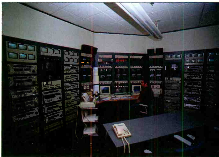
This master control room is capable of originating up to 10 channels of on-request pay-per-view programming with only one operator.
