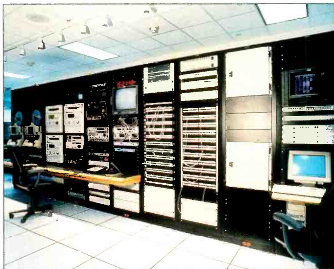
The central control room provides full support for the compression suites. The room is equipped with a serial digital router, digital and analog videotape machines for master tape playback, and full machine control capability.
