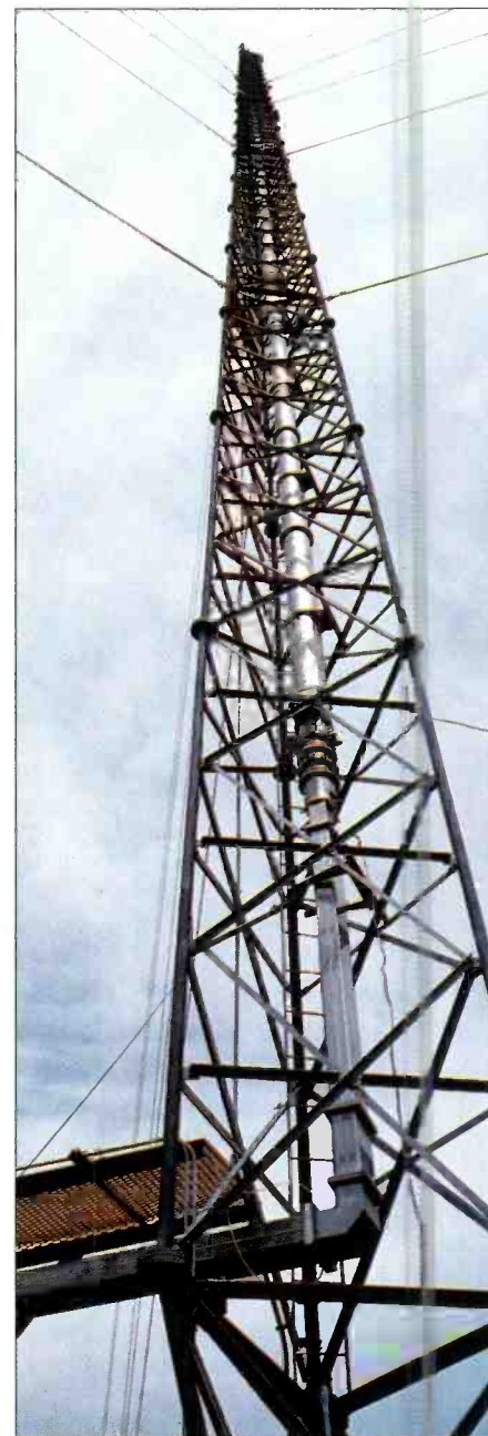
This high-power UHF-TV transmission line uses circular waveguide.
