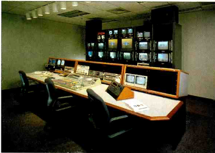
Typically, production control rooms are not included as part of an automation system, however, portions can easily be automated if desired. (Photo courtesy of Bill Straus Photography, Inc.)
