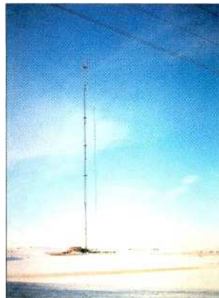
This 1,430-foot tower located on property owned by the University of Wisconsin currently holds three TV, three FM and numerous smaller antennas. The design provides for additional antennas to be added later.
