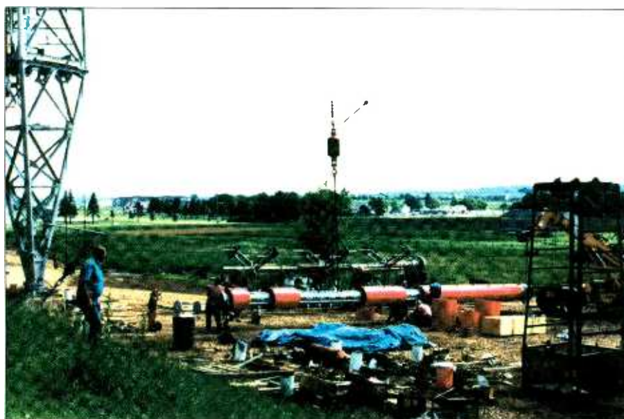
On the ground, WISC's (Channel 3) antenna was stacked on top of WHA-TV's (Channel 21) antenna. (Photo courtesy of Ken Dixon.)
