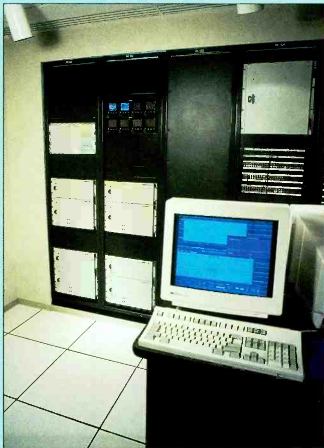
The Home & Garden Television network became a beta site for the BTS Media Pool service shown above. Combining the video server with a robotic tape system, provided the network with on-air reliability, operational flexibility and the ability to adapt as new features and technology become available.
