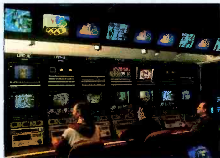
NBC's New York edit control room, located at 30 Rock.
