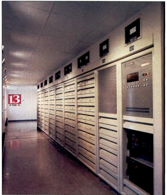
WTHR's new Harris HT 70HSP transmitter.
