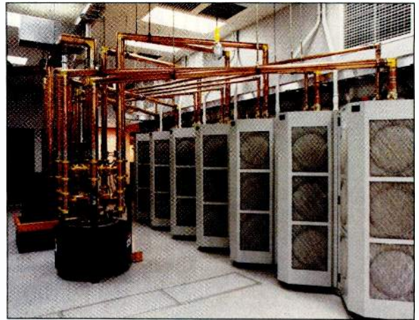
New Harris seven-way, high-power Geysel combiner.
