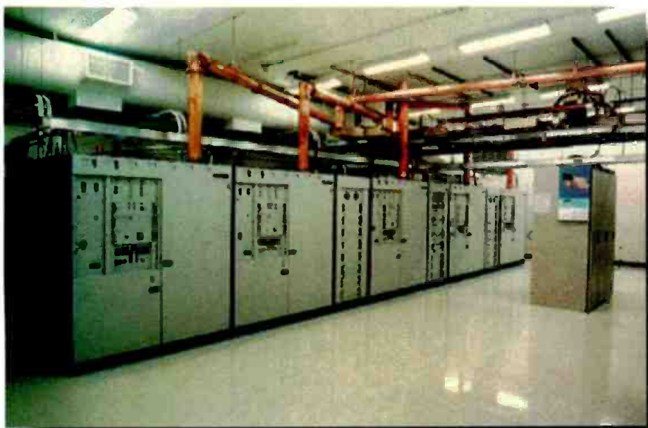
The Comark "IOX" transmitter installed at WXIN, Indianapolis.
