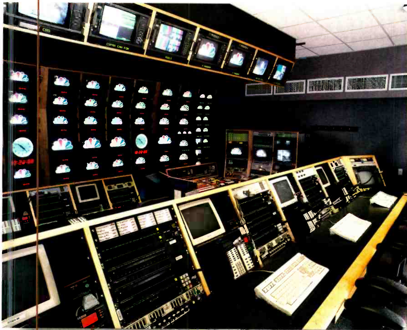
With a large infrastructure of NTSC and a November deadline, the networks are faced with a huge challenge in converting their facilities to HD in a short timeframe. Shown here is an NBC news control room in Washington, DC. Most stations will initially have to rely on NTSC-to-HD upconverters to generate high-definition signals. (The NBC facility built by and photo courtesy of Communications Engineering Inc., Newington, VA.)
