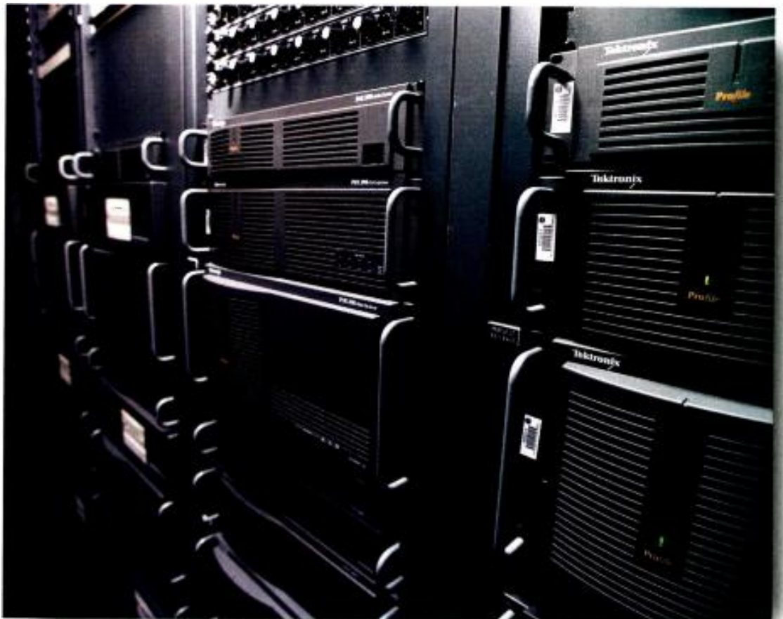
Digital storage is centered around 12 Profile PDR200 video file servers, linked to dual Silicon Graphics Origin 2000 servers. Total capacity is 1.44TB.
