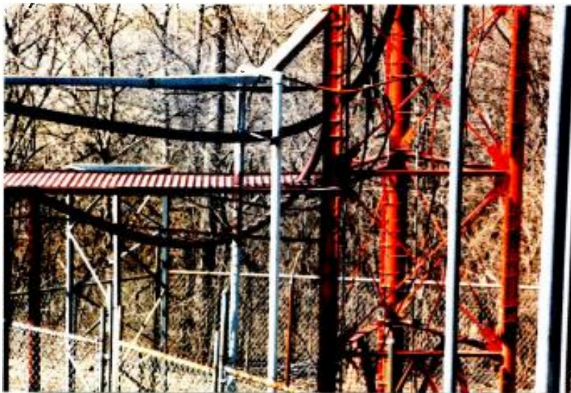
When using semi-flexible transmission line, care must be taken to support the line and observe the minimum bending radius.
