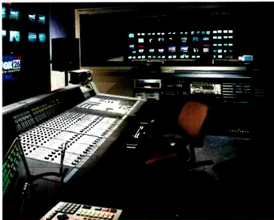
Photo: The recently installed audio control room at KRIV, Houston, was designed by DTA Carlson, Chicago. (Courtesy Aker/Zvonkovic Photography, Houston)
