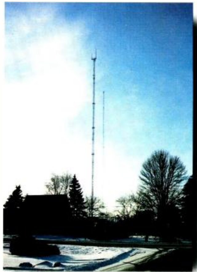
A variety of details must be covered when planning multi-station towers and facilities, including antenna and transmission-line placement, as well as dividing the costs among those involved.
