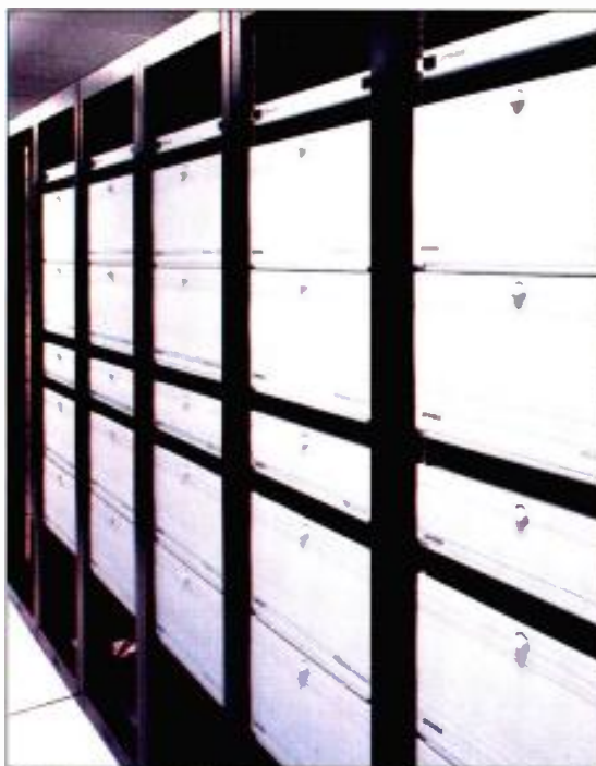
The Pro-Bel HD series routers occupy only five racks, yet provide 160 crosspoints.
