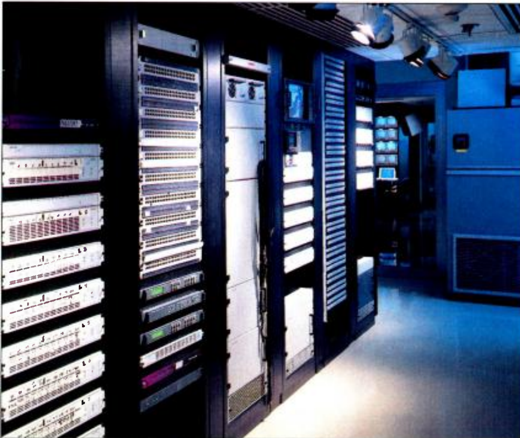
Rack room showing distribution amps, patch panels and a Leibert computer room air conditioning unit in the background.
