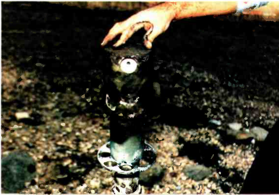
A conductive path can form as dust, dirt and moisture accumulate within a transmission line. When that path arcs over, the ultimate result is transmission line failure.
