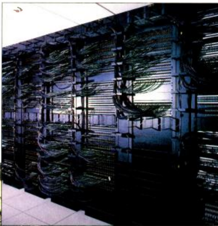
The unique application of coaxial and twisted pair Icon modules in the central equipment room (above) and at remote demarcation locations (photo left), provides KCET with an extensive pre-wired cable trunking system to support rapid system changes and upgrades. Top photo by Sandra Williams.
