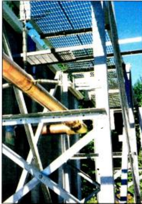
Proper installation of rigid transmission line includes the use of appropriate hangers along both horizontal and vertical runs.
