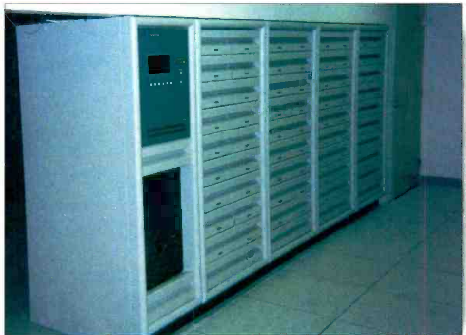
The Harris PT40CD DTV transmitter at WPLG-TV, Miami, gives 40kW peak and 10kW average power.
