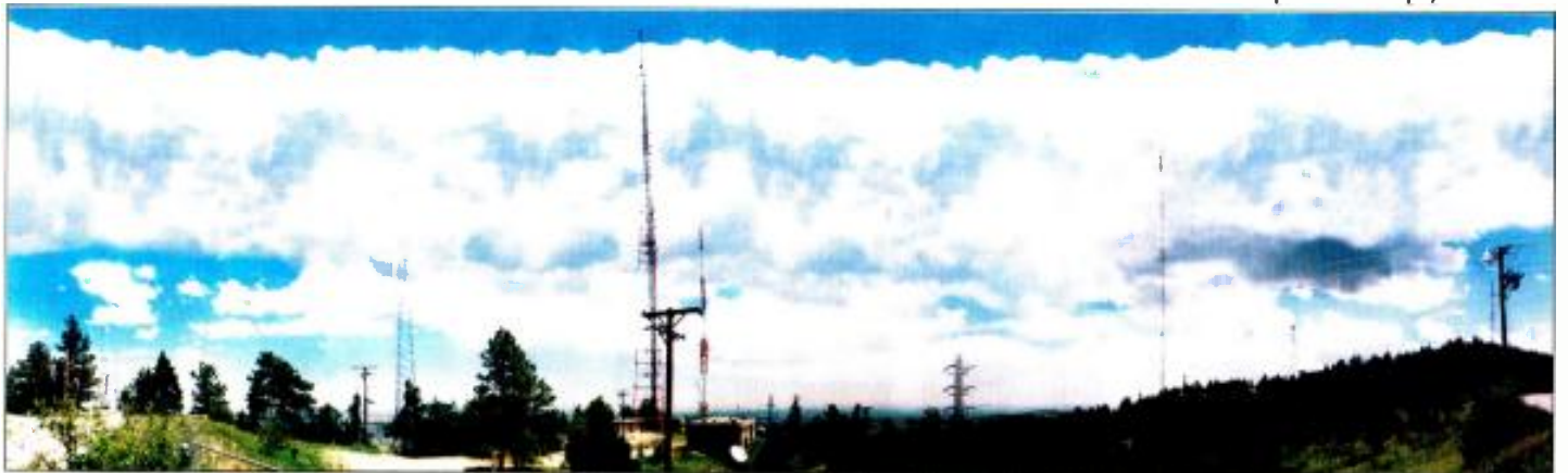
Seven Denver television stations have their broadcast towers and antennas located at nearby Lookout Mountain. A coalition of five stations faces opposition to its plan to build a single DTV tower and remove existing NTSC towers. Photo provided by Virtual Topics Inc.
