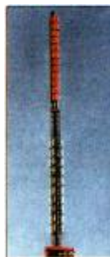
Dielectric Stacked antennas
