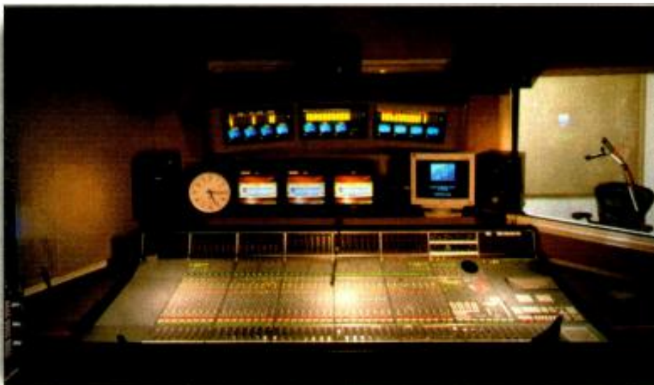
The Times Square Studios facility features a Solid State Logic 48-fader Aysis Air digital broadcast console. (Photo courtesy Solid State Logic. Photo by Dave King)
