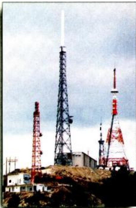
DTV Utah's transmitting facilities on Farnsworth Peak near Salt Lake City include a 330-foot tower. Currently, two of the eight consortium broadcast stations are transmitting a digital signal.
