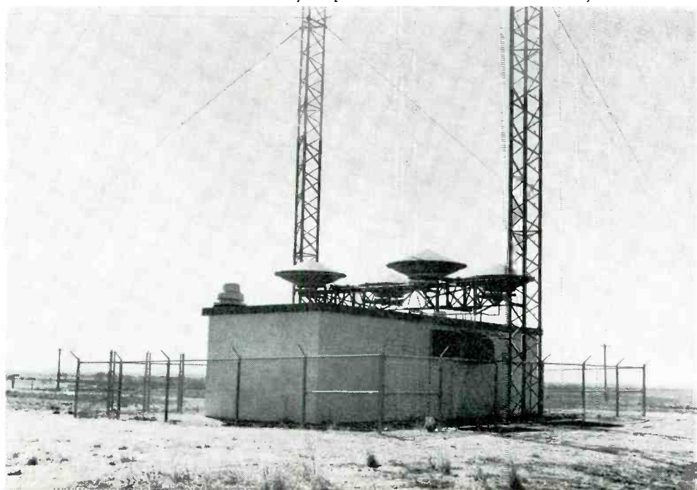
6000-MC Two-Way Repeater with Dual Path Diversity.
