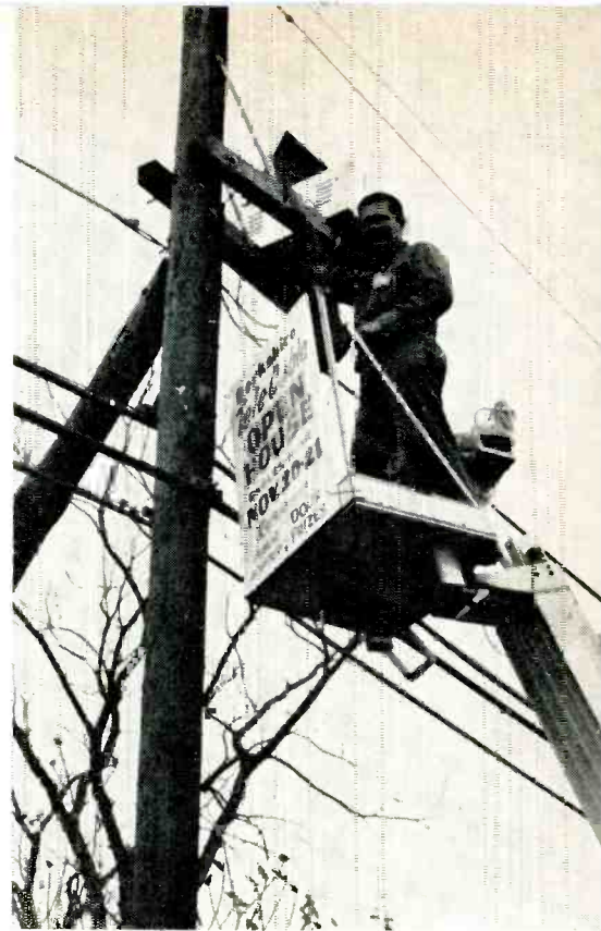
Berkshire technicians like Roy Mannikko use Uti-Lift for maintenance of amplifiers where feasible.
