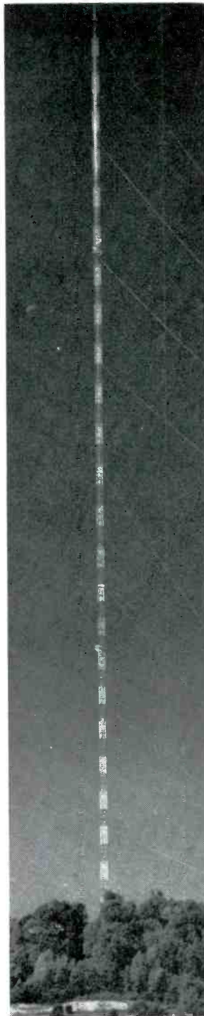
WBIR-TV, Ch. 10, Knoxville, Tenn. Tower Height: 1,750' Visual ERP: 316 kw Grade A Coverage: 9,850 sq. mi. Total TV Homes: 292,300 ARB Net Weekly Circ: 216,200 Tower Facility Cost: $580,000
