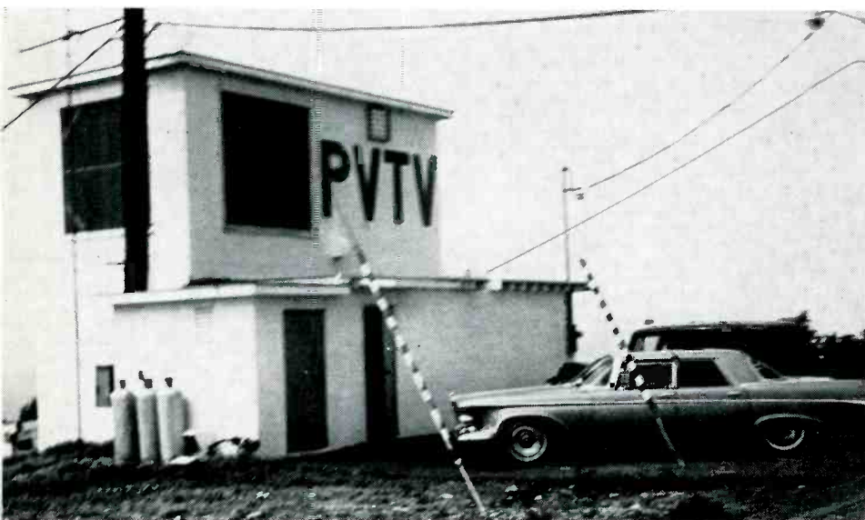
This two-story, masonry-block structure is located atop one of the highest ridges in the area, approximately 2,000' above sea level. It houses the head-end and microwave receiving equipment. PV's small but modern and efficient closed circuit studio is also located in a partitioned off section. This site also serves as a microwave relay station for Potomac Valley Telecasting Corp. The dark panels in the second story level protect the microwave dishes.
