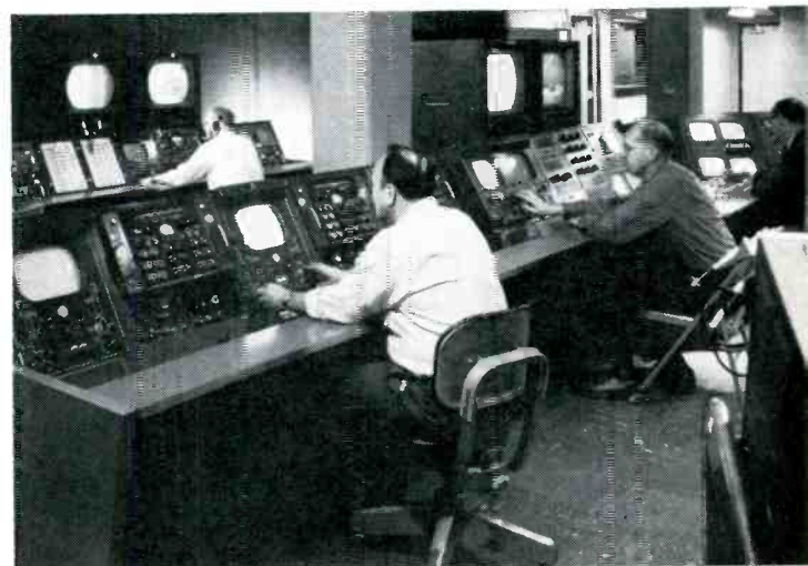
WHDH-TV Master Control. At upper left is video control for live color studio programs. Film camera video control at lower left. Far right is master control operation.
