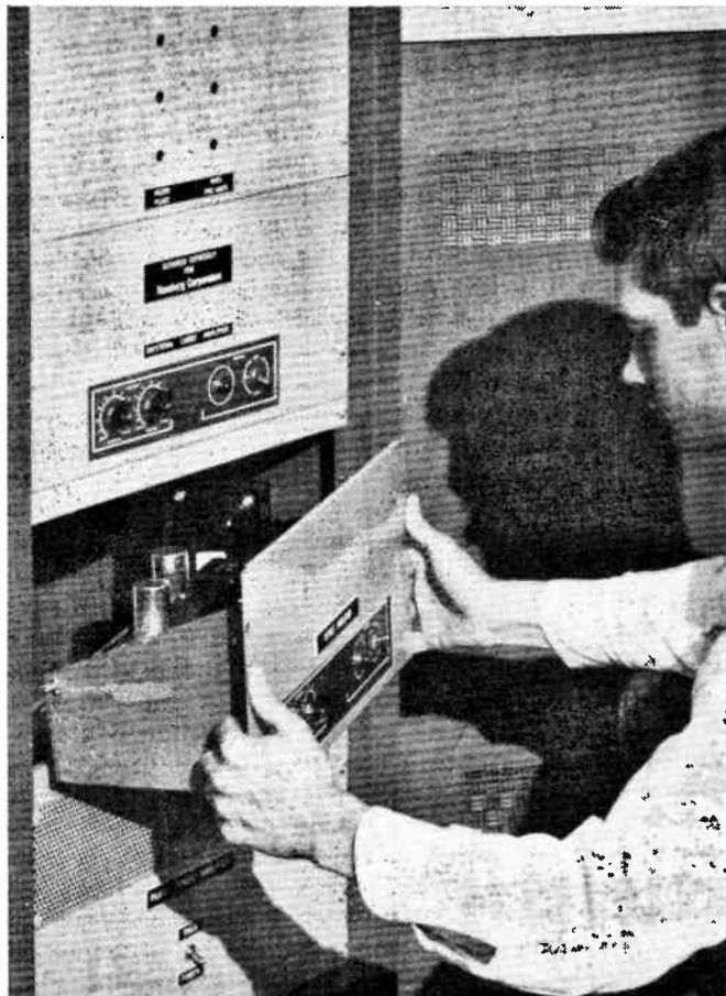
Bennie Colyer installs one of three power amplifiers in an industrial sound system equipment rack.
