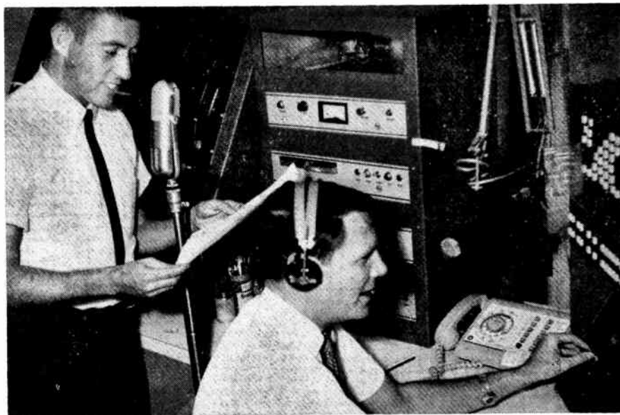
Production Director Dave Archard (seated) and announcer Jim Howell shown recording commercial in WFUN's production room. Buttons above the control board operate various audio circuits, including a reverb, equalizers, filter, an Ampex 350 and two 354 tape machines, and two RCA cartridge machines with record. Custom-built equalizers and Hammond reverb can be switched in for special effects and equalizing.
