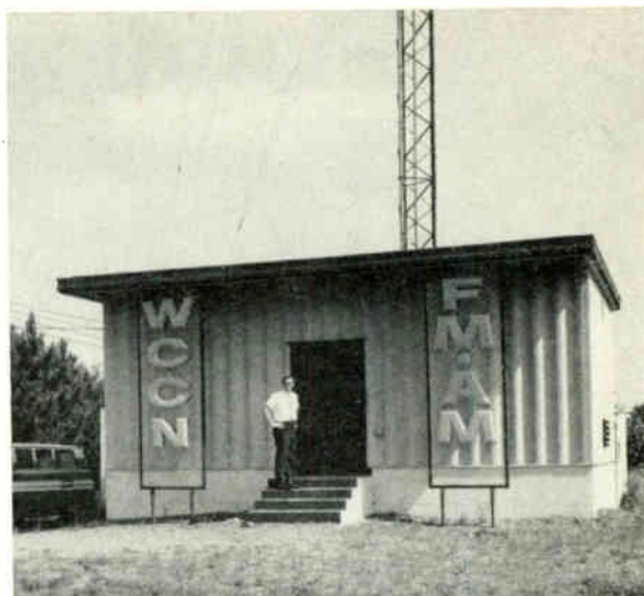
Building on Neillsville's north side, made of Bethlehem steel with copper screen under entire floor structure. Arc lamps on roof light tower structure at night.
