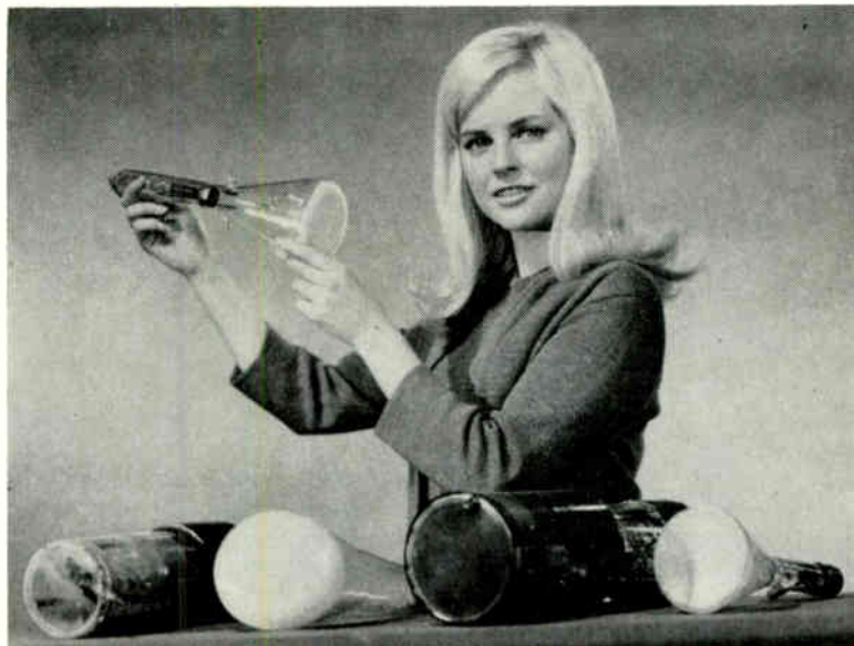
Dr. Philo T. Farnsworth's tubes, dating from 1927, include, left to right on the table, the first image dissector, first projection oscilloscope, a primitive image orthicon with electron multiplier and the first oscilloscope tube with a flat screen. Victoria Lynch of ITT holds the world's first oscilloscope with internal deflection plates.
