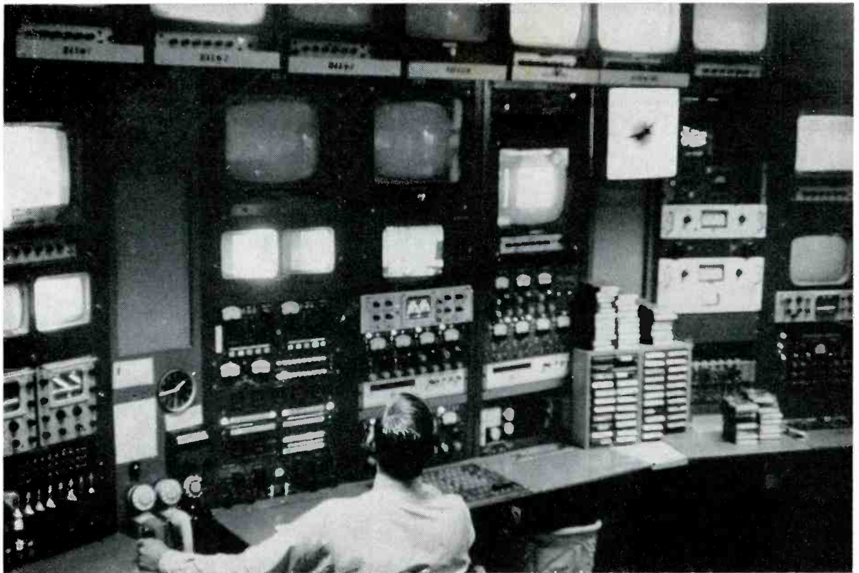
Master control for two TV channels is a hodgepodge of added-on gear and can select any source for either channel.
