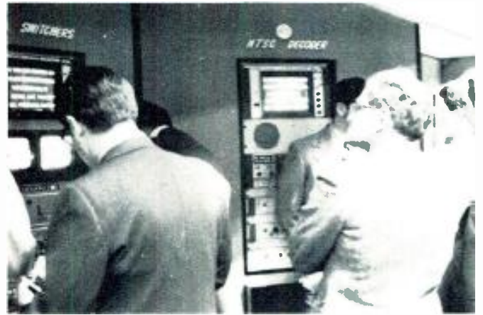
Telemet had a new NTSC decoder.
