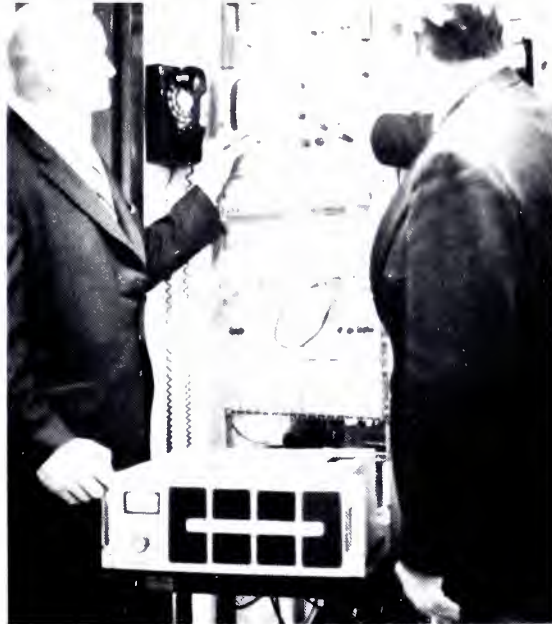
Anderson and Paulson (TMI) checking TBC output.
