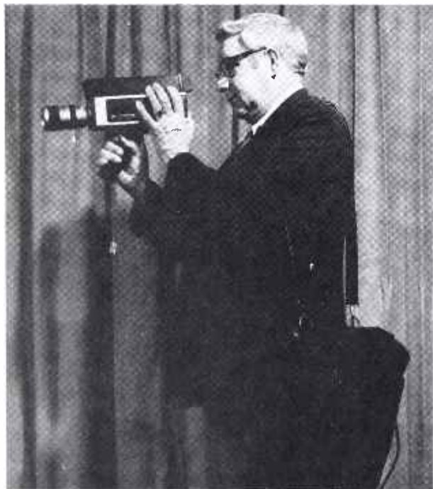
Magnavox Chromavue 440 is one of the portable video cameras newly on the market which are getting tryouts for some areas of television news gathering. Others are listed in box on earlier page. Such portables will ordinarily involve a backpack with the electronics for the cameraman, plus a VTR carried by a second man or in accompanying mobile unit.
