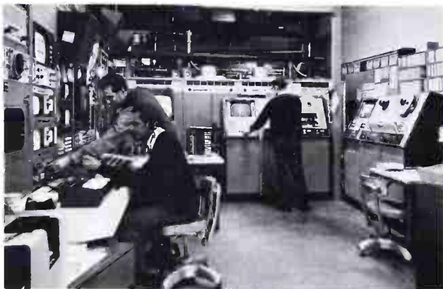
Control area at KBMA-TV includes master control, left, VTR's in background.
