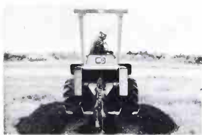
Double-auger digging assembly.
