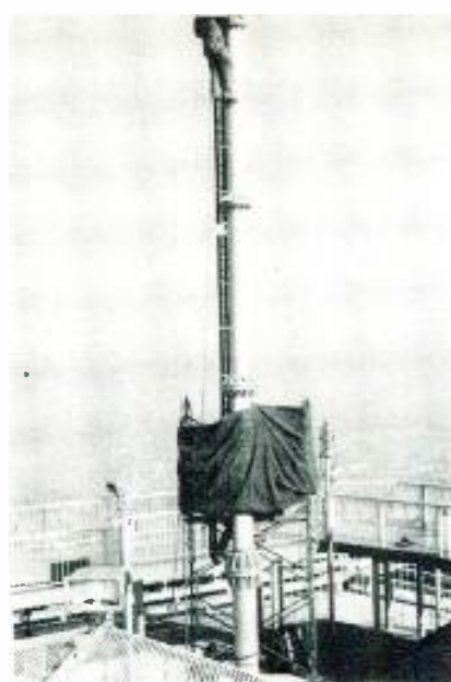
At New York City's World Trade Center, ABC goes full speed ahead with its CP installation, remaining convinced of CP's benefits
