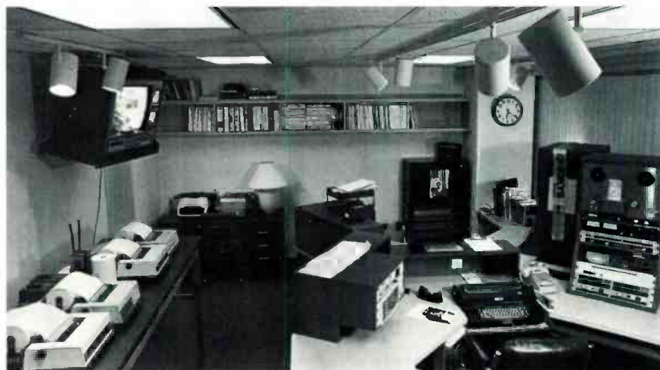
One of three work stations in the newsroom shows the Farrtronics intercom and two-way control (left) and turret with Utah Scientific routing switcher and tape players on the right.
