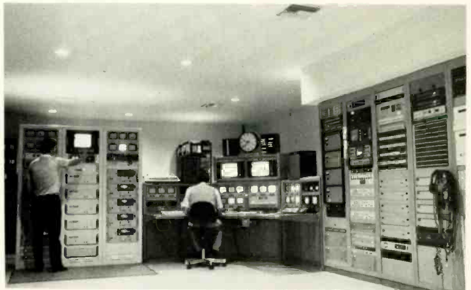
Master control includes the Lake Systems La-Kart II system, the key to KSCH's automation.
