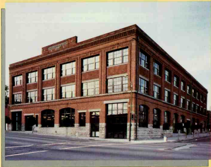
San Francisco headquarters of Dolby Labs is based in a renovated 1910 brick building.
