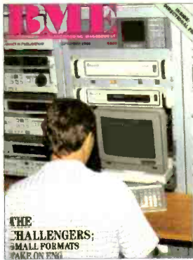
On the cover: S-VHS control system at KCCO/KCCW, Alexandria, MN.
