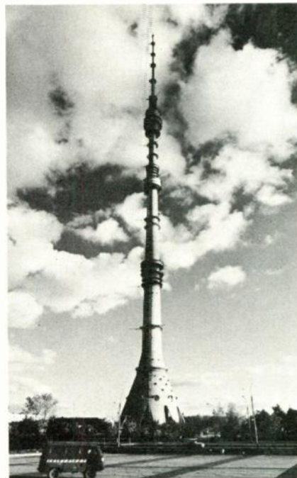
In the late afternoon sun, Ostankino Tower reaches toward the clouds with its 533-meter (1748-foot) high TV mast. It will be the key relay point for television images and sound from the Moscow Games that will blanket the rest of the world.
