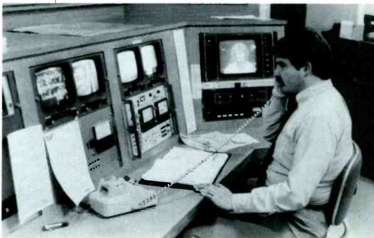
The ENG control area for Gannett affiliate KPNX-TV in Phoenix is capable of receiving three simultaneous satellite feeds.
