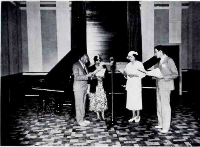
THE NEW ORGAN STUDIO AT WBEN , BUFFALO, N. Y. VELOCITY MICROPHONE SHOWN IN FOREGROUND, AND ORGAN SWELL-SHADES IN BACKGROUND
